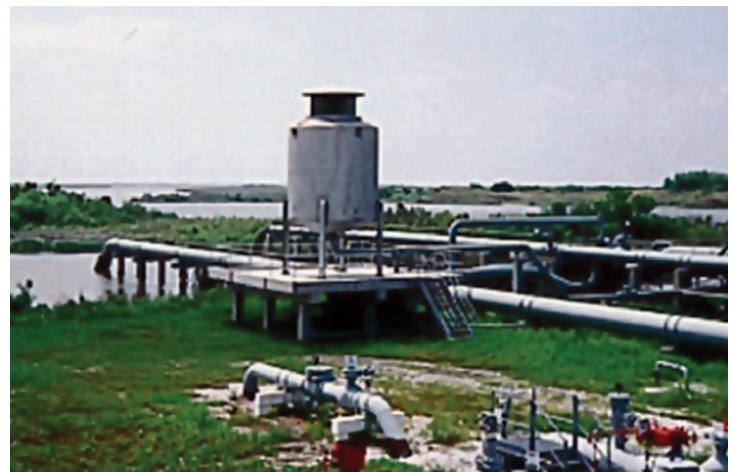
All stainless steel construction BDSS for wetlands application.
