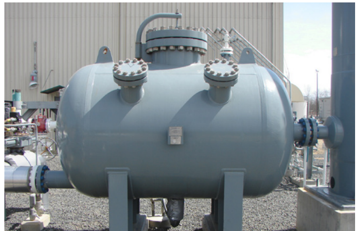
Typical stationary CB carbon bed blow down vent deodorizer configuration.
